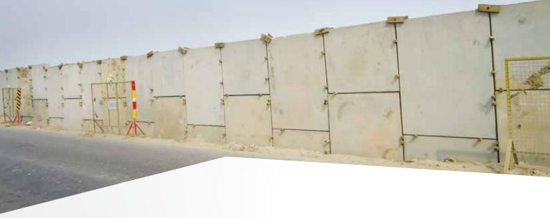
StrataWall™ is a precast concrete panel wall fascia for a reinforced soil structure. StrataWall™ is designed to give a positive concretion with StrataGrid™ geogrids as a reinforcing material.
