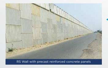
StrataWall™ panels are either T-shaped or Square reinforced concrete panel fascia, each about 3 sq.m., for a reinforced soil structure. The reinforced soil structure is a mass of non-plastic soil which is reinforced by StrataGrid™ geogrids.
