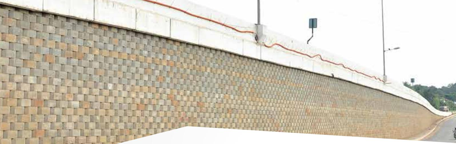
StrataBlock™ is a modular precast concrete block fascia for a reinforced soil structure. The reinforced soil structure is a mass of non-plastic soil which is reinforced with StrataGrid™ geogrids. The concrete used is plain cement concrete of M30 grade which gives high durability.
