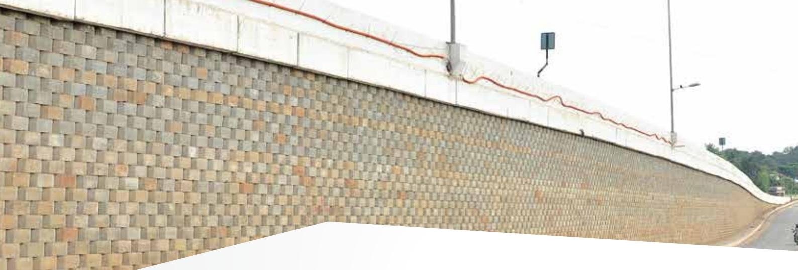
StrataBlock™ is a modular precast concrete block fascia for a reinforced soil structure. The reinforced soil structure is a mass of non-plastic soil which is reinforced with StrataGrid™ geogrids. The concrete used is plain cement concrete of M30 grade which gives high durability.
